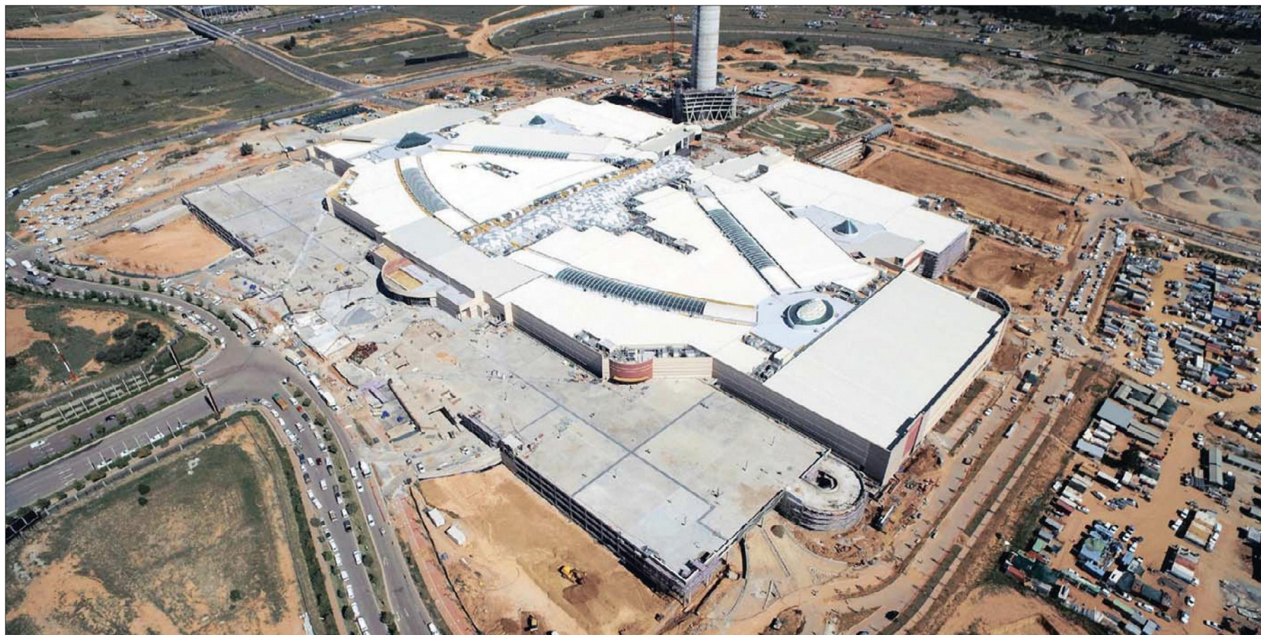
The Mall of Africa situated between Pretoria and Joburg opens to the public this week.
