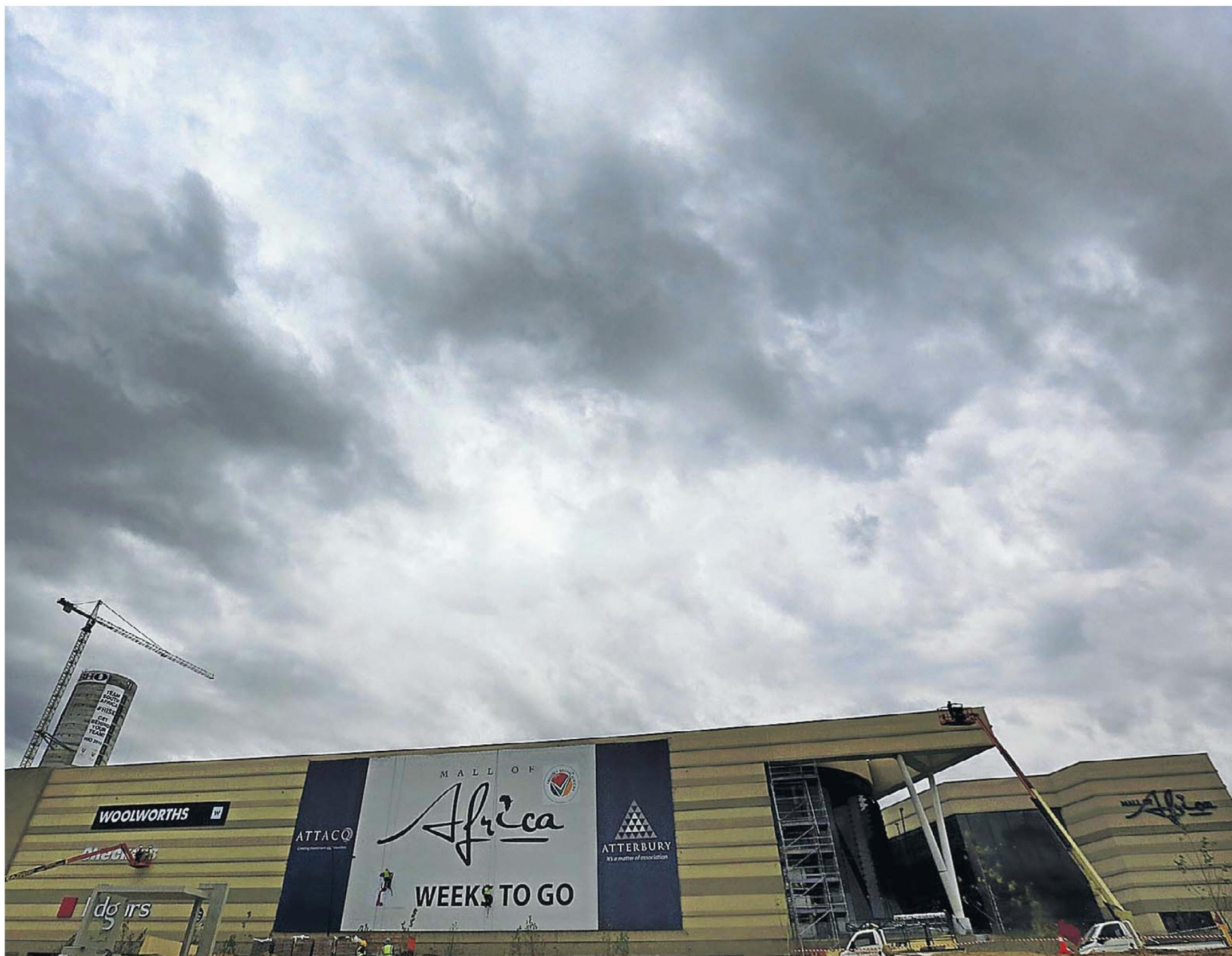
BUSY: Construction workers move up and down the facade of the Mall of Africa in the last week before it opens to the public on Thursday. The mall, in Midrand, has more than 300 shops and will be the largest on the continent to be built in a single phase Picture: SIZWE NDINGANE
